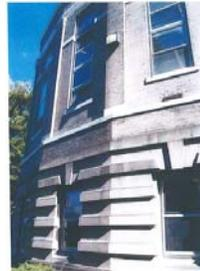
Floor of building showing upper windows. It is the upper portion of the rear exterior that is in critical need of rehabilitation due to rusting steel beams.
